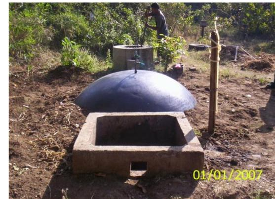
Replacement of brick work dome by Polyethylene dome – savings in time & energy for installation
